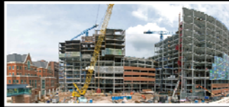
Construction Progress in October 2008
